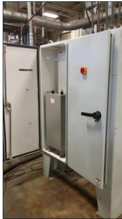
**Figure 6. NEMA 12 Cabinet Housing the Components of the Power Supply (the main capacitor is shown)**
