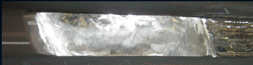
Step 4: Grinding preparation for taper-fill layer
