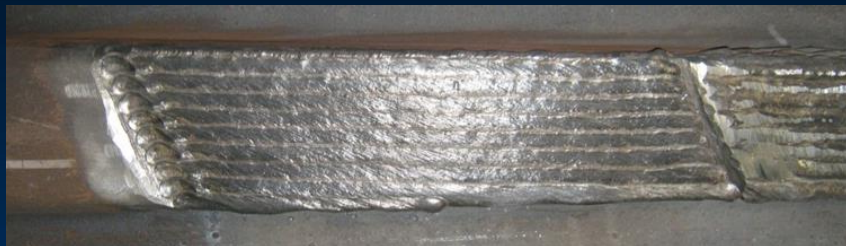
Step 5: Welding of taper-fill layer
