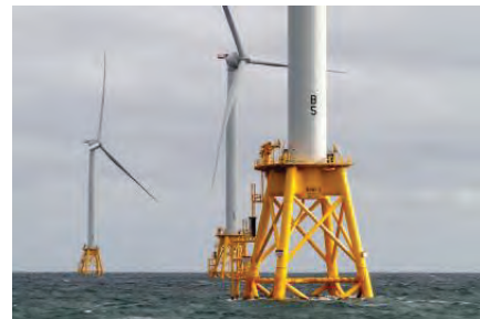
Block Island Wind Farm (Rhode Island)
