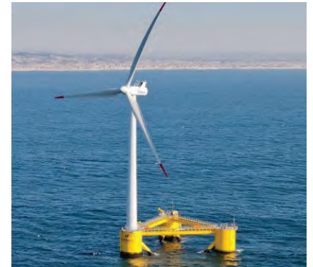
Principle Power's Windfloat Design
